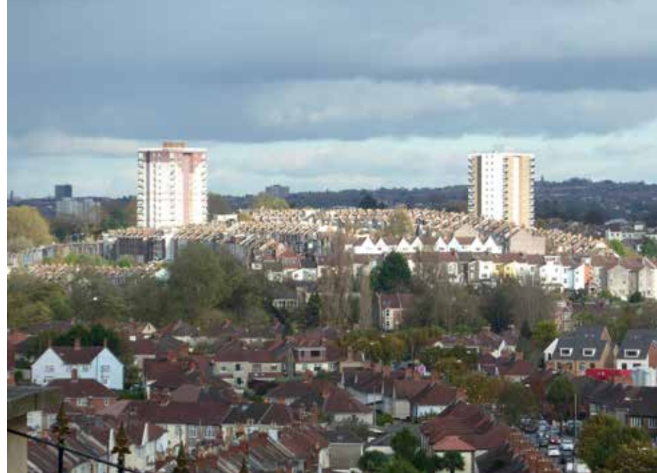
Above left, Polden House and Holroyd House, Windmill Hill. Above right, Gilton House, Brislington.
