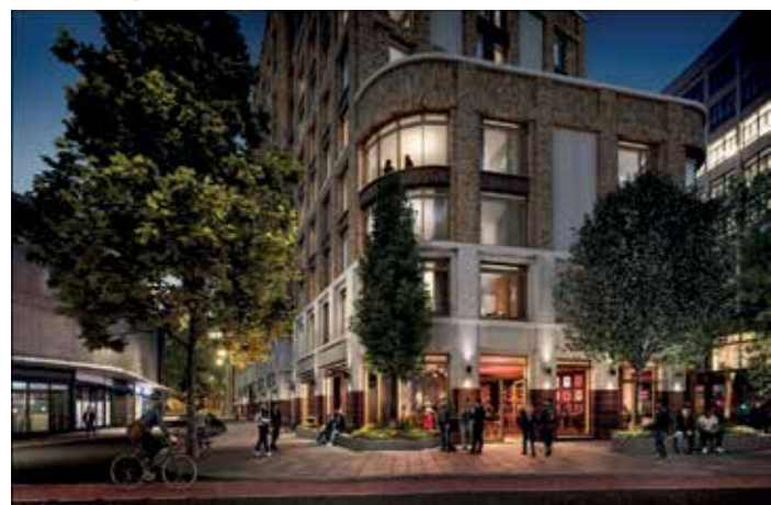
Fairfax Street. Nice entrance but too high.
