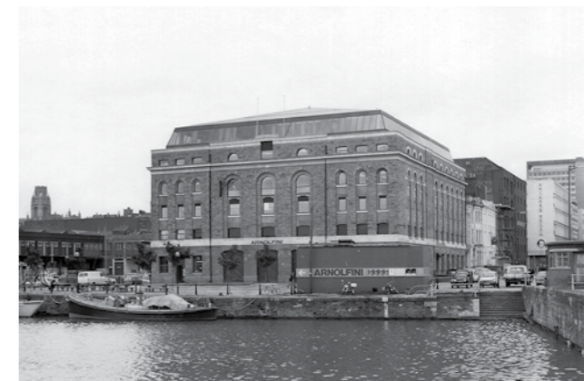
Above left, Bush House, one of the best known buildings on the harbourside.
