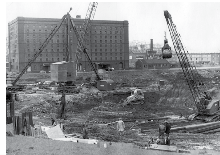
Foundation work for the Ashton Pumping Station exposed an old river quay seen in the foreground. In the background is A Bond Warehouse. Photo taken on 3 April 1968.
