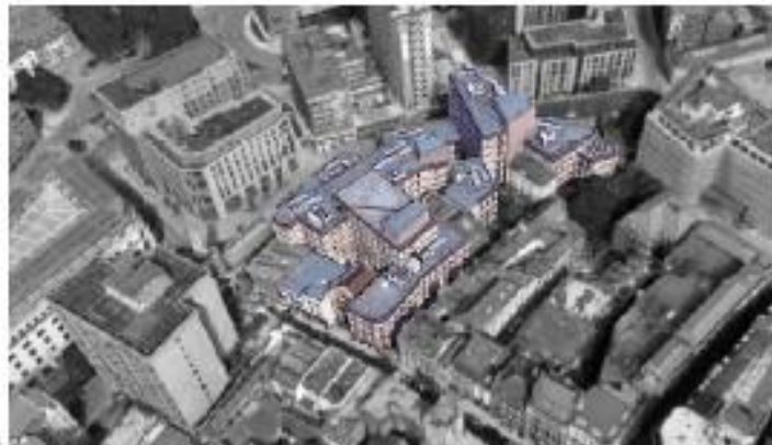
Construction of NatWest Court
