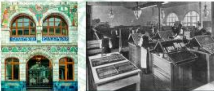
Construction of Everard's Printing Works
