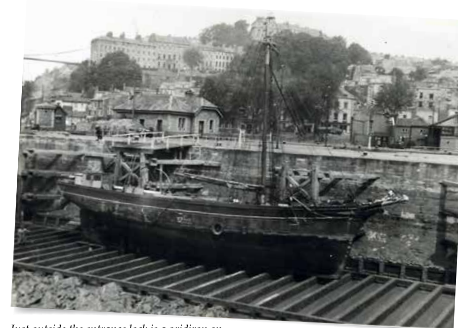
Just outside the entrance lock is a gridiron on which ships were placed to allow minor maintenance.
