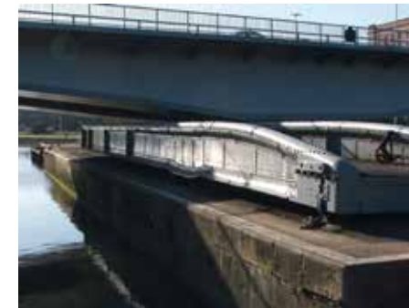
Brunel designed a swivelling bridge to cross his new entrance lock.
