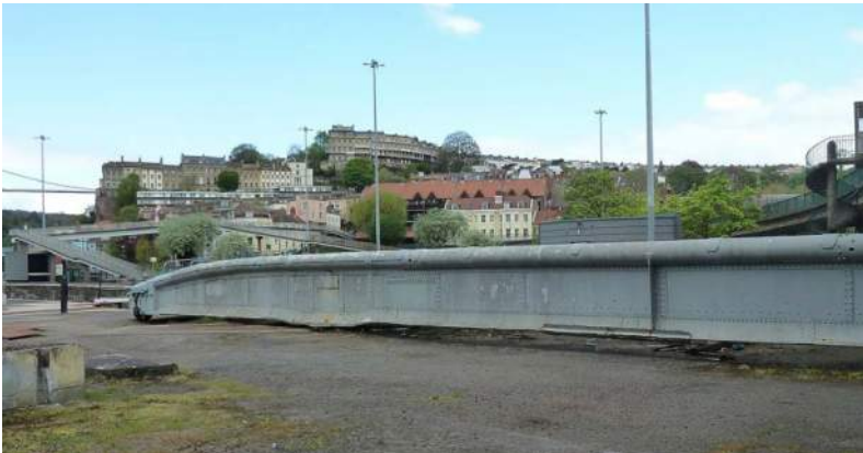
Brunel's tubular wrought iron bridge. By Andy Dingley - Own work, CC BY-SA 3.0,
