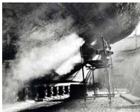
Above, Some of the earliest conservation work; high-pressure water blasting on the hull, 1971 (© Colin Momber)
